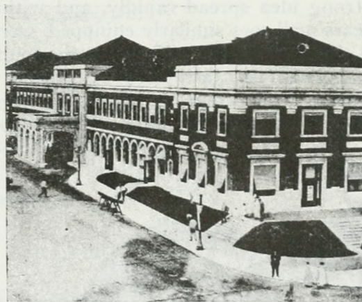
A MODERN PASSENGER STATION—The Illinois Central station at Champaign-Urbana is designed to provide the maximum of comfort and convenience to the traveling public. Thousands of university students use this station each year.
