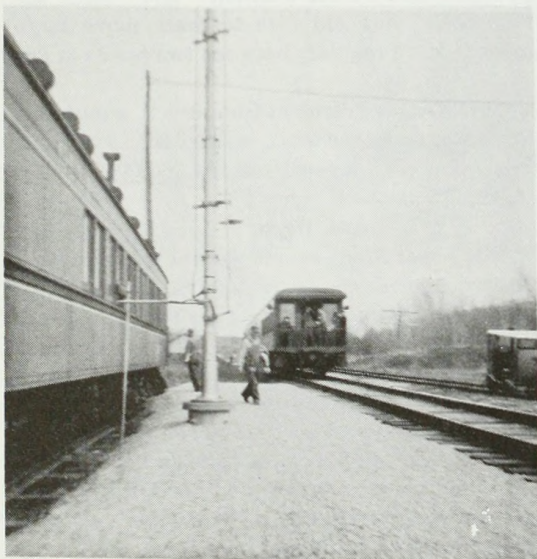
.....Pulling out of station for last time
