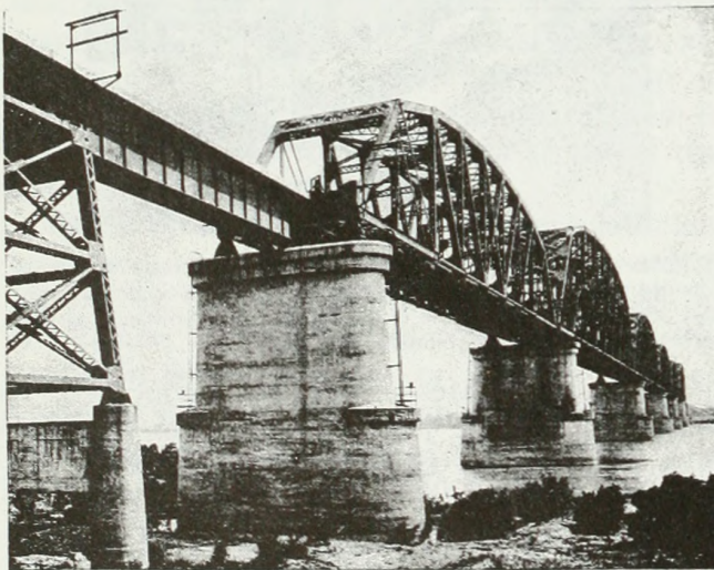
A MAJESTIC RAILWAY BRIDGE—At Metropolis, the site of old Fort Massac, landing place of the first Americans to establish their homes in Illinois, this great structure of concrete and steel spans the Ohio River, forming one of two routes of the Illinois Central between Chicago and New Orleans. The other and older route is through Cairo.
