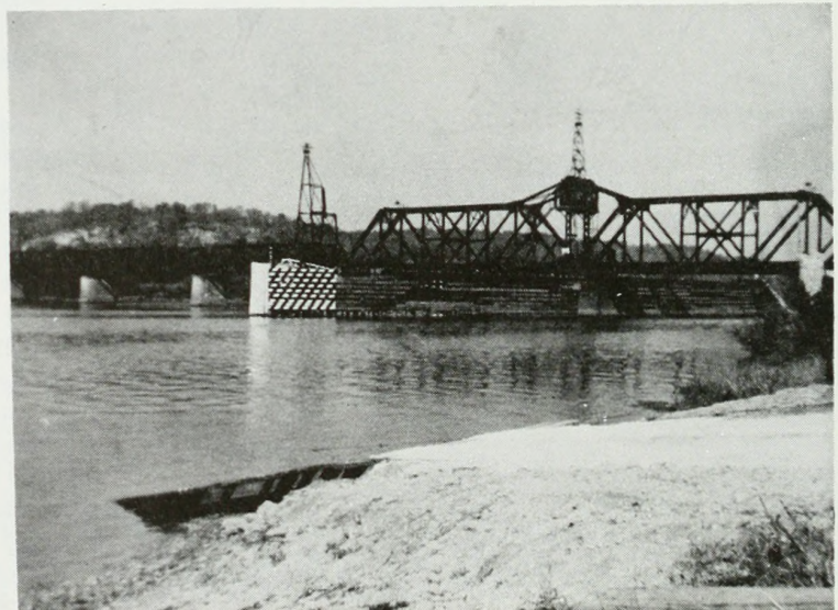
....Illinois River Bridge at Pearl
